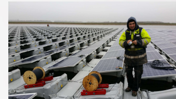
Junction Box Cabling
