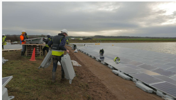
Structure assembly and PV cabling on platform
