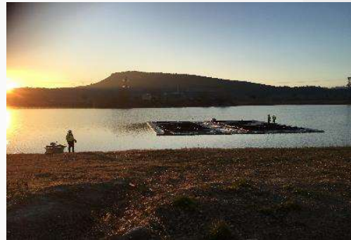
O'MEGA 0.2 28 kWp Piolenc, France
