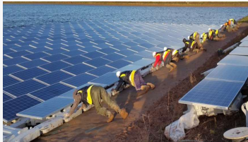
Substructure launching on platform
