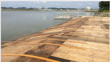
Launch platform installation
