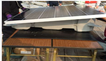
PV installation on floats
