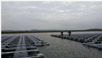
Sub-structure offshore assembly
