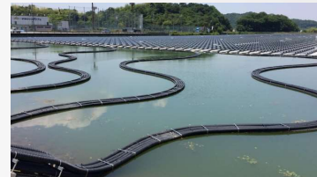
Cabling to the shore
